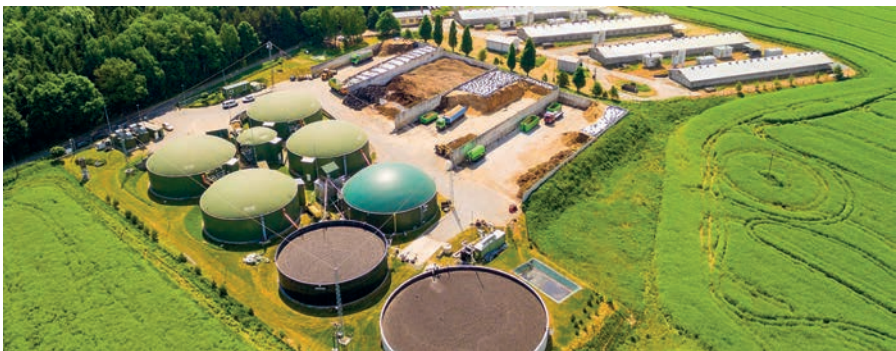
Figure 4. Biomass power plant (Energy Power Plant, 2022).
