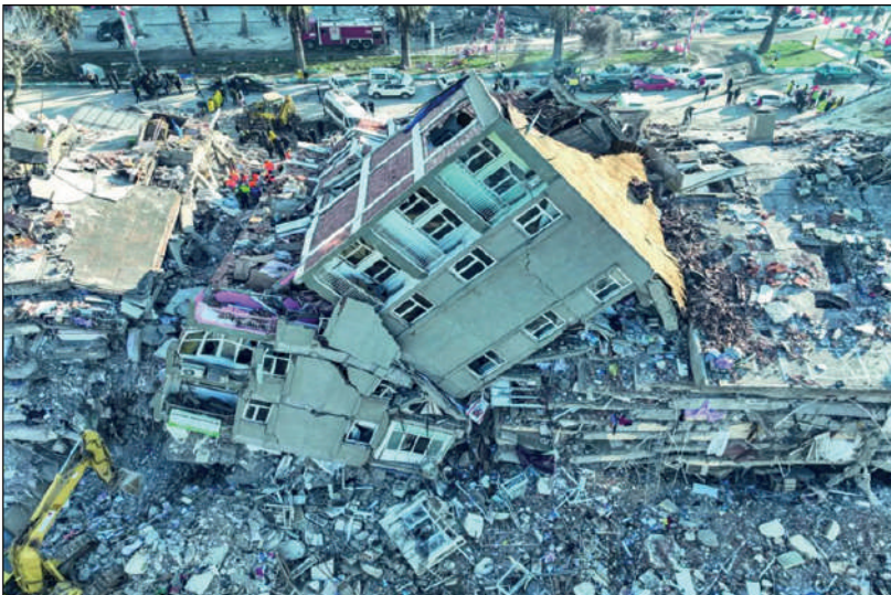
Figure 26 : Collapsed Buildings in the Kahramanmaraş Earthquake: Consequences of Illegal and Non-Standard Construction
